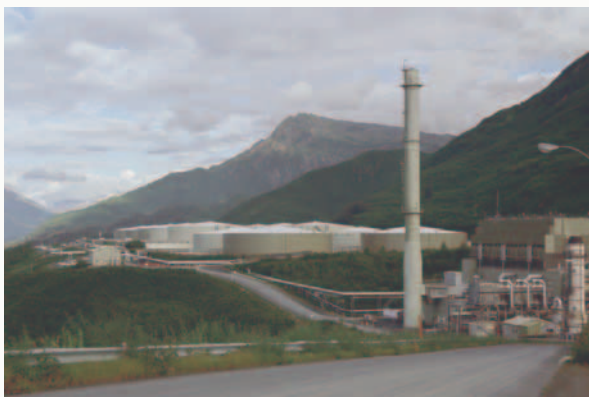
18 holding tanks contain 9.18 million barrels
